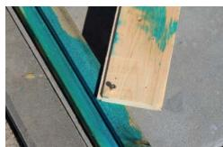
Lay out the base frame on your foundation as shown in the drawing. Lay it out so that the door is located at the desired position. Screw the frame together beginning at the corner opposite the door. Make sure the corner is at a right angle. To keep the corner from moving, screw a board (leftover pieces from the package) opposite the corner on the upper edge of the frame.
