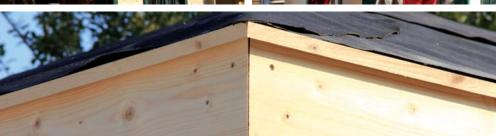
Attach the pre-cut fascia boards all around with screws to the tops of the rafters. Make sure they are flush at the corners (dimensions in the drawing).
