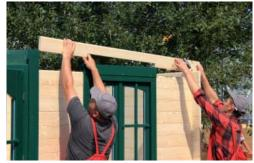
The final rows exceed the door area and have to be firmly connected. (*It may help to use a large screw clamp.*) Screw the corner above the door together from above and below.
