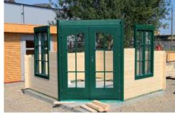
Now complete the walls according to the drawing and always check the number of wood profile rows to be built.
