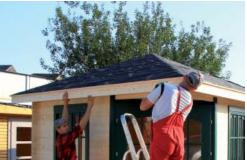
As the last step, lay a square piece of roof felt centred over the top and attach it.
