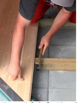
Begin laying the foundation beams. Lay them as shown and dimensioned in the drawing into the floor and attach the foundation beams with screws to the frame.
