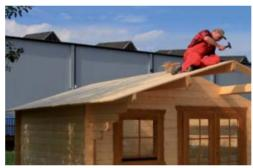
Now mount the **gable boards** at the front and back. Fix the gable boards with screws to the roof boarding and the ridge/centre purlin; the spacing between the upper edge of the gable board and the upper edge of the roof boarding should be approx. 5-6 cm.
