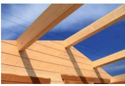
Insert the two centre purlins into the slots in the gable. Make sure the beams (purlins) are flush and at the same angle with the gable. Adjust them with a hammer if necessary. Now set the second (smaller) piece of the gable between the two centre purlins and on the already assembled front part of the gable. Repeat this step for the rear gable. Then insert the ridge purlin into the upper slots of the gable.
