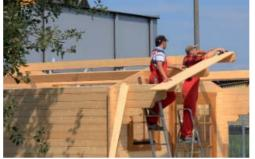
Now nail the boards twice to the ridge/centre purlin and the fascia board. Lay the roof boarding all the way to the back. Measure in regular intervals to ensure that they are properly aligned and that the spacing to the wall is consistent. The backmost (final) board needs to be cut to size in most cases. Afterwards, mount the remaining boards on the other side as described above.
