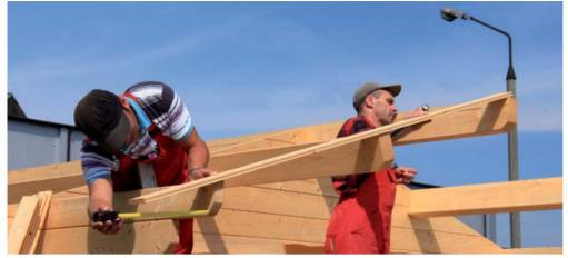
The roof boarding is already cut to the correct length so that you only have to lay the boards from front to back.
