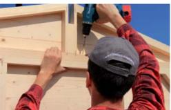
Use a wooden board to protect the gable elements against hammer blows. This will help you attach the gable element firmly to the wall element. Screw the gable elements and the wall elements together properly.
