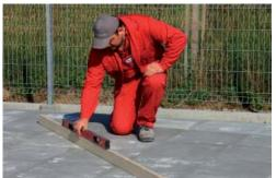
As a basic principle, only build your summer house on a level surface. Check your foundation prior to assembly!
