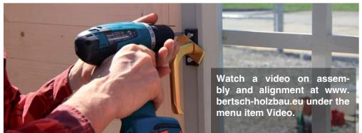
Insert the window handle into the lock in the window. Use a cordless screwdriver or a screwdriver to screw in the uppermost screw.
