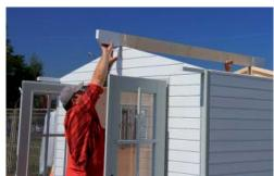
Now place the ridge purlin in the prefabricated slots. Attach the two fascia rails on the left and right hand-side of the gable.
