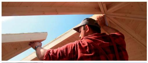
Now take a screw clamp and tighten the adjusted roof element at the roof overhang (outside) and screw them together from the left and right handside. Place two small pieces of wood underneath the clamp to protect the wood.
